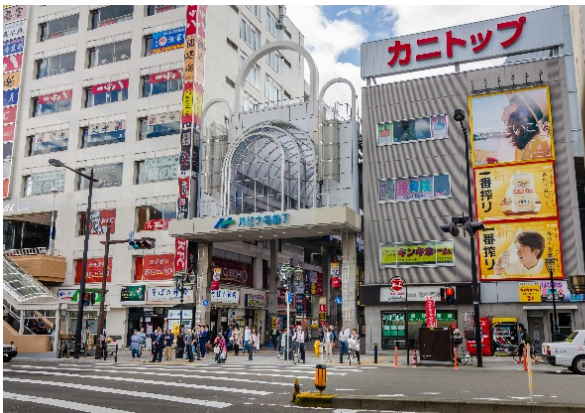
Entrance to Sendai Japan arcade complex: on the left is escalator to railway station and elevated walkway
