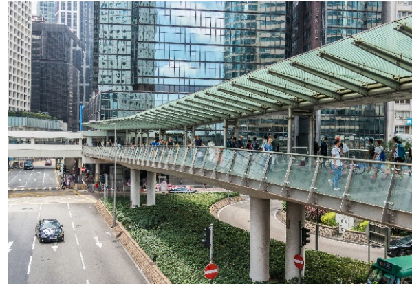
Hong Kong elevated walkways network, the roof provides shelter from rain and sun; Bangkok has now adopted this kind of network
